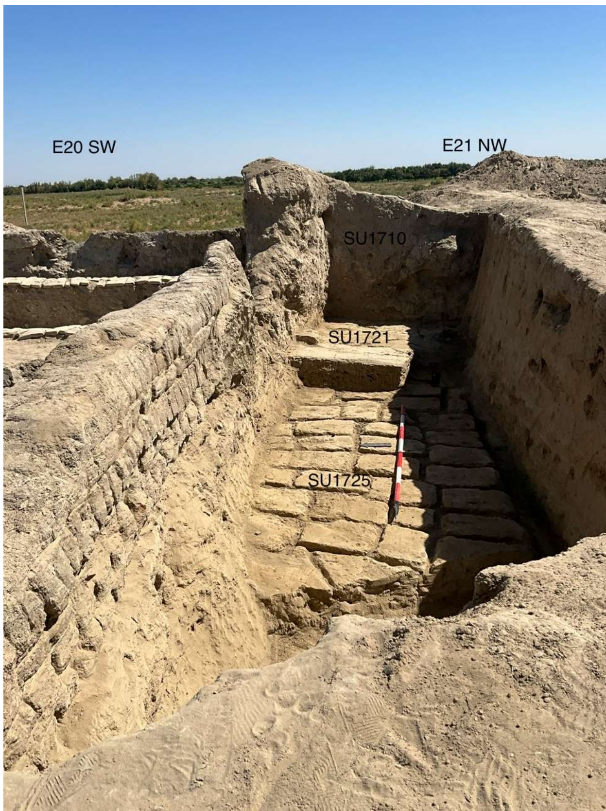
FIG. 14 Trench E21-NW: shahristan wall 1710=91; mud bricks, part of the sealing platform (SU1725) (view from W).
