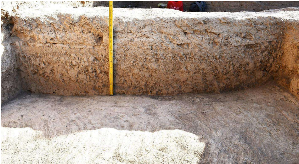
Fig. 36. R-3. North wall of room 5, view from the south
