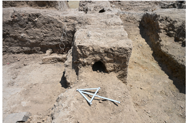
Fig. 16: Detail of doorway elements
