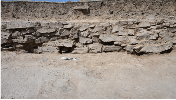
Fig. 20: Stone wall from the front view.
