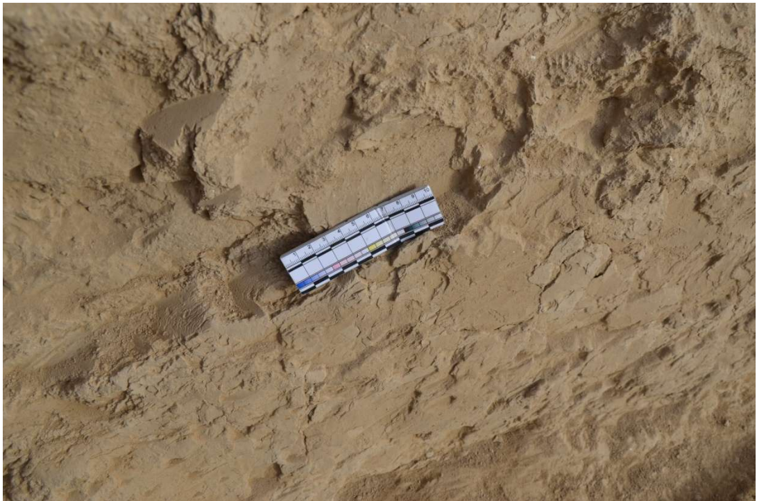
Figure 146. Element 23. Fragment of the inner surface of the northern wall from the second and third construction periods, with preserved plaster and traces of sealing. Top view to the north.
