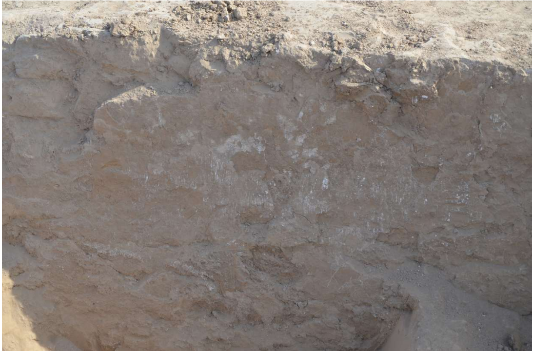
Figure 115. Element 12. Fragment of the internal surface of the eastern wall from the second and third construction periods, with preserved plaster and traces of whitewash. View to the east.
