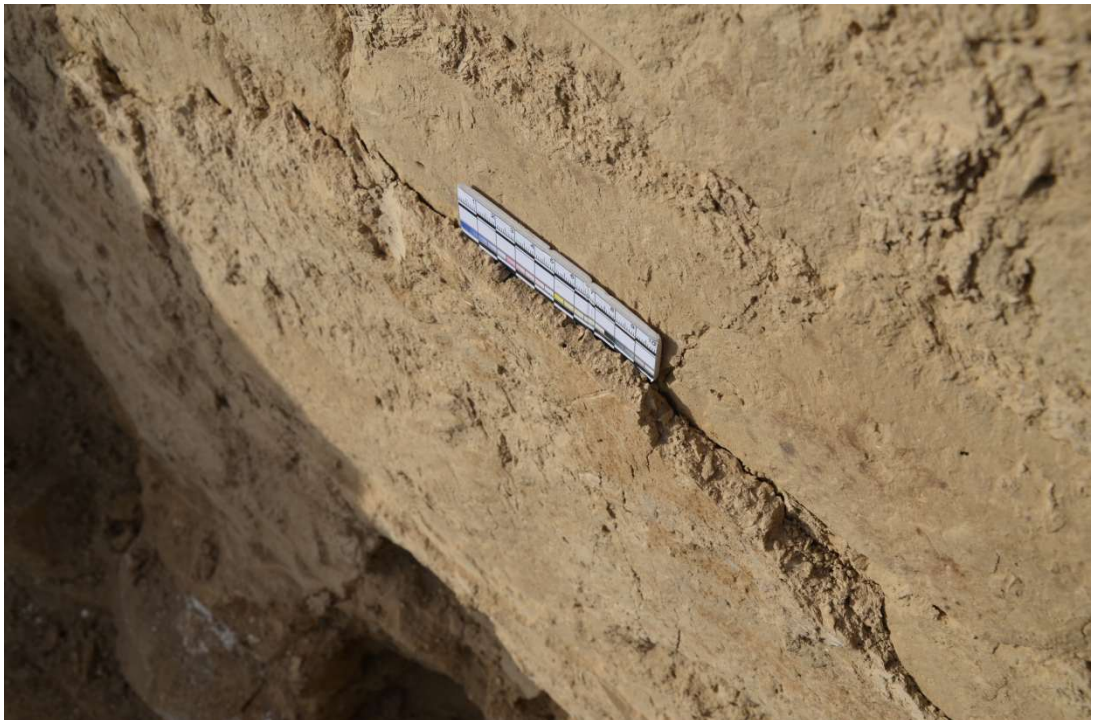
Figure 148. Element 23. Fragment of the inner surface of the northern wall from the second and third construction periods, with preserved plaster and traces of sealing. Top view to the north.
