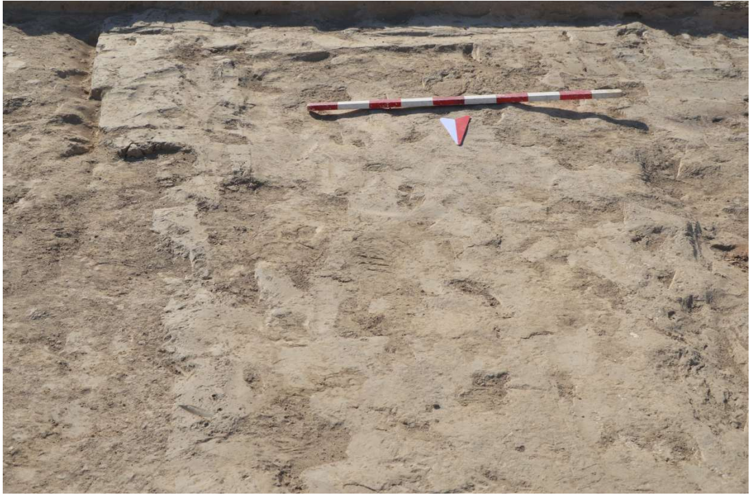
Figure 103. Element 11. South wall of the late construction period. View to the south.
