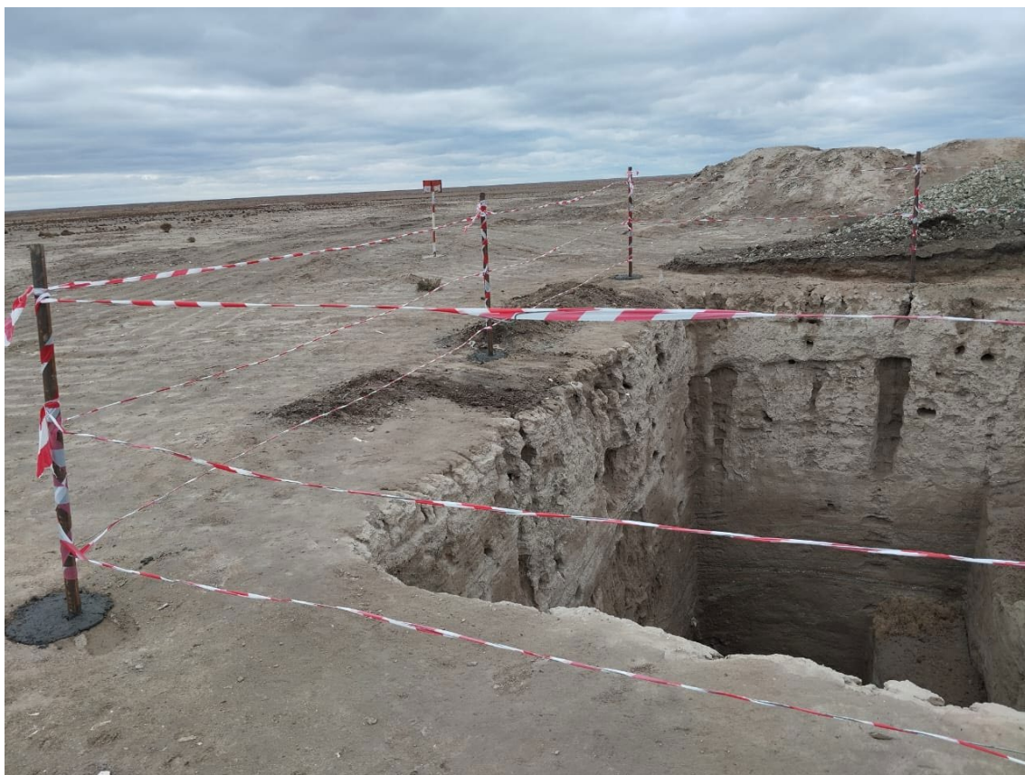
Figure 28. Installation of fencing around the excavation after completion of work.
